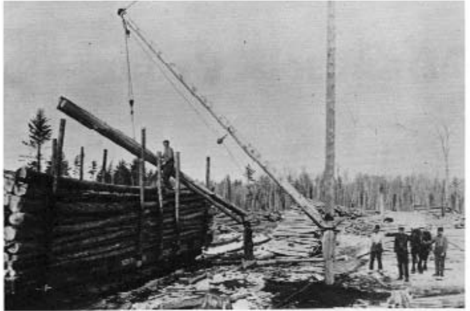
Below: Loading cedar on flat cars with sawing boom "jingle." Center: A water tank on an ice road. Bottom: two-bank drey for skidding posts to logging roads.
