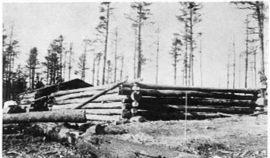
Most early camps were made of logs, as this one under construction.
