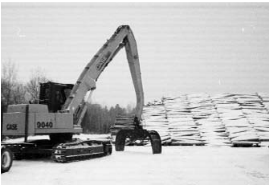
The loader and the beginning of the piles to be covered in sawdust and frozen.
