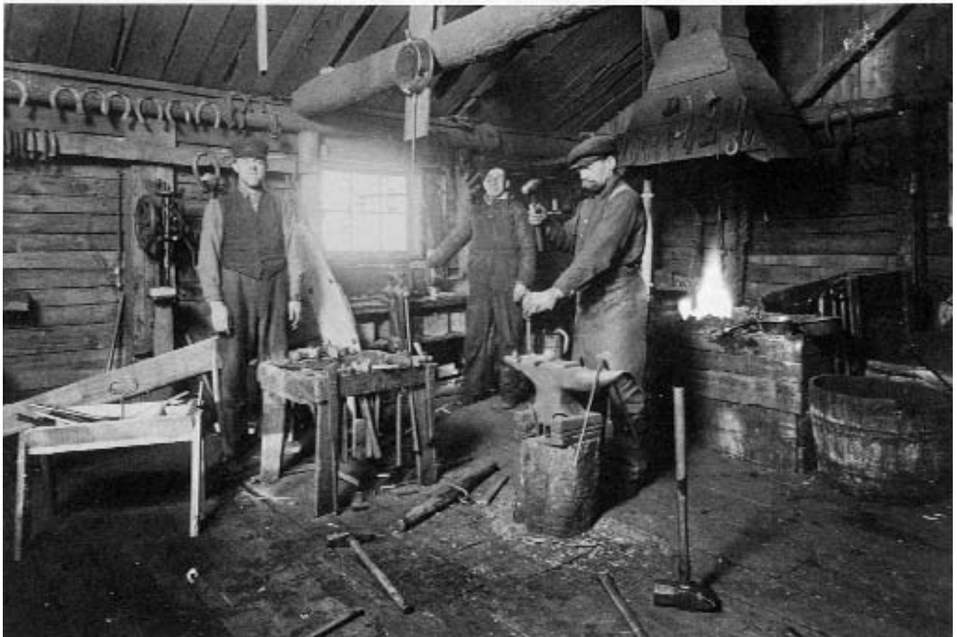
Smith, in typical apron, and heavy men at Golbroth & Co. Camp No. 4 in 1912. Back barrel by forge was for tempering
